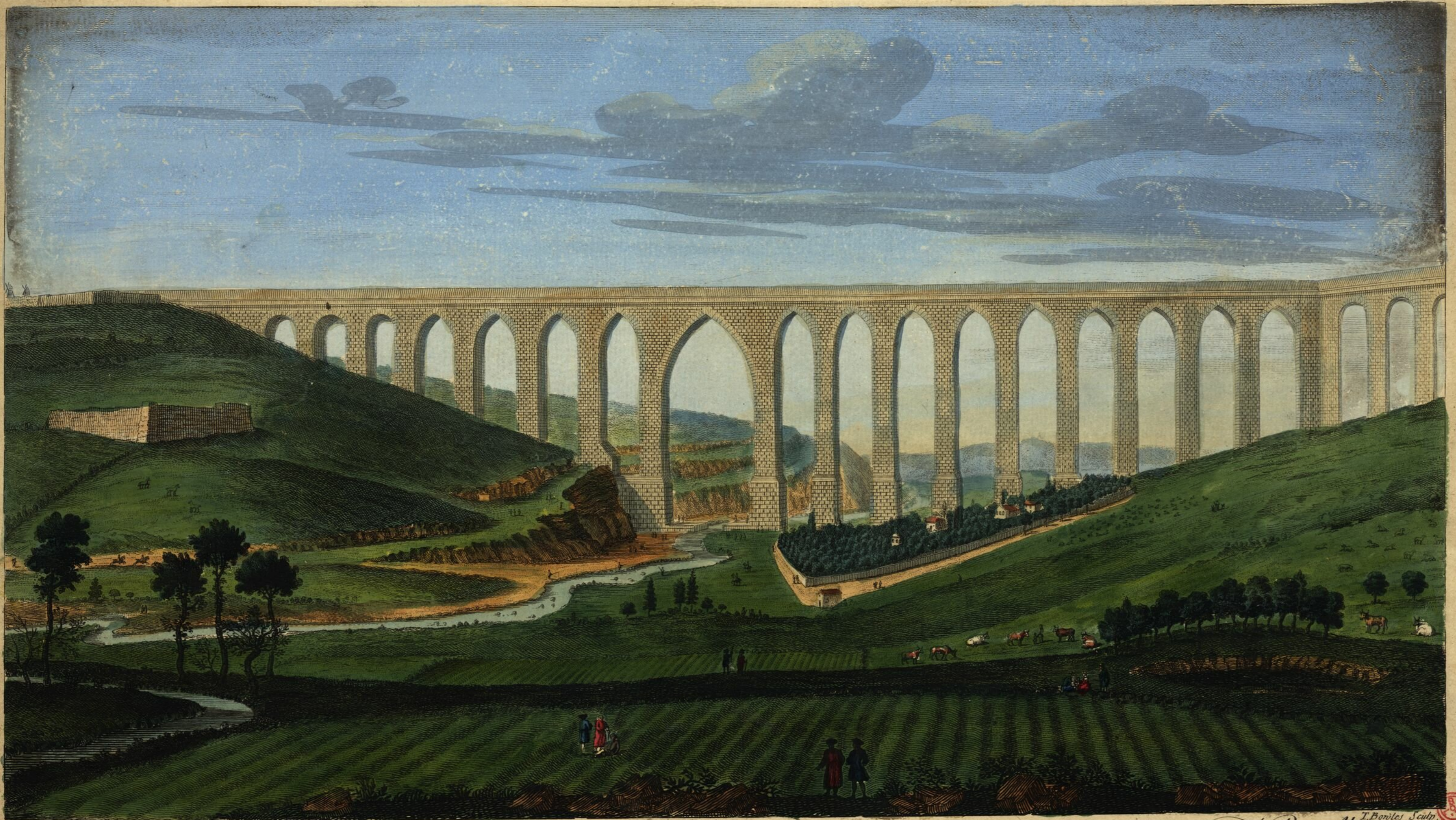
R. Black delin. A PROSPECT of the new Aqueduct of Lisbon, as Crossing over the Valley of Alcantra on Stone Arches, the Largest of which is 150 feet wide, and 249 feet High. Which is 47 feet higher than the Monument in London. T. Bonito Sculp. PERSPECTIVA dos Novos Arcos d'Agua que a travessem o Val de Alcantra, altura do Mayor Arco he 332 Palmos, e a largura he 200 Palmos. London Printed for Rob. Wilkinson, 58 Cornhill.
