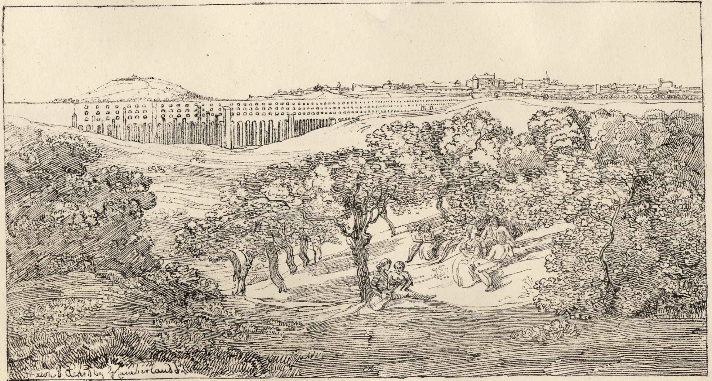
A View of Elzas with the Aqueduct and Fort La Lippe.
